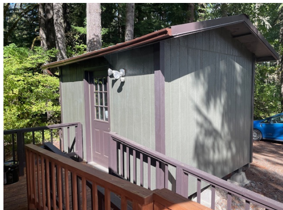
Library Annex building with new gutters
