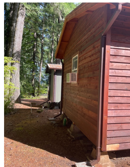
Side of main building with new gutters/downspouts
