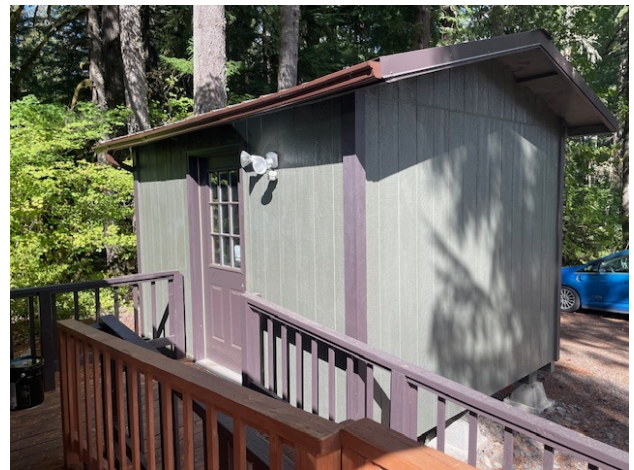
Library Annex building with new gutters
