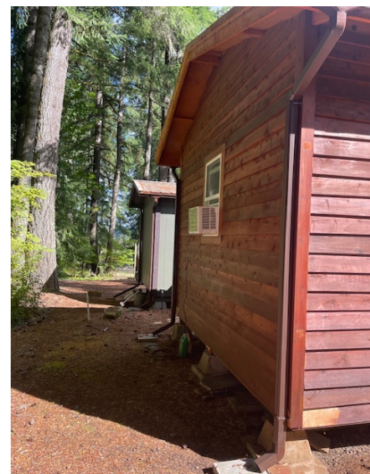
Side of main building with new gutters/downspouts
