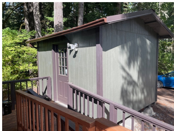
Library Annex building with new gutters
